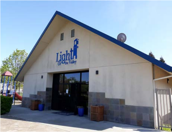
Light of the Valley Church – front entry
