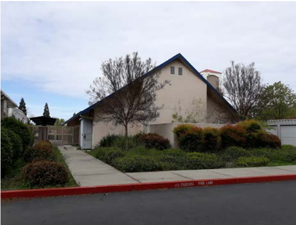
Looking north at rear elevation of church
