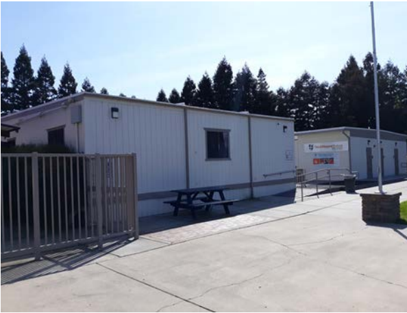
North side of the Classroom Buildings
