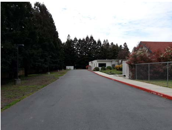
West view of the fire lane on south side
